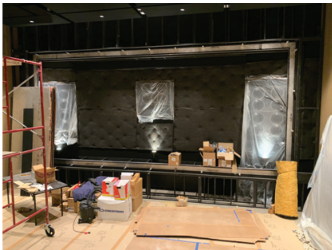
PMC LCR's mounted behind the 22-foot screen.
